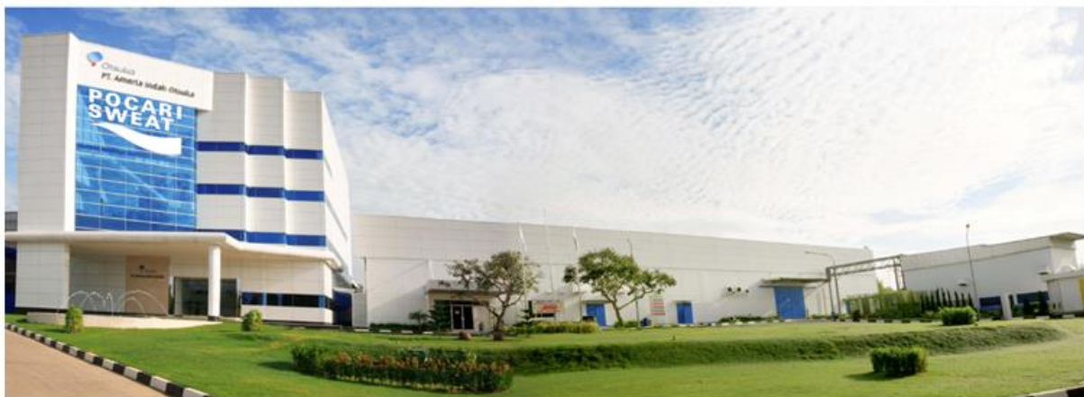
Sukabumi Factory ORONAMIN C DRINK production facility (exterior view)
